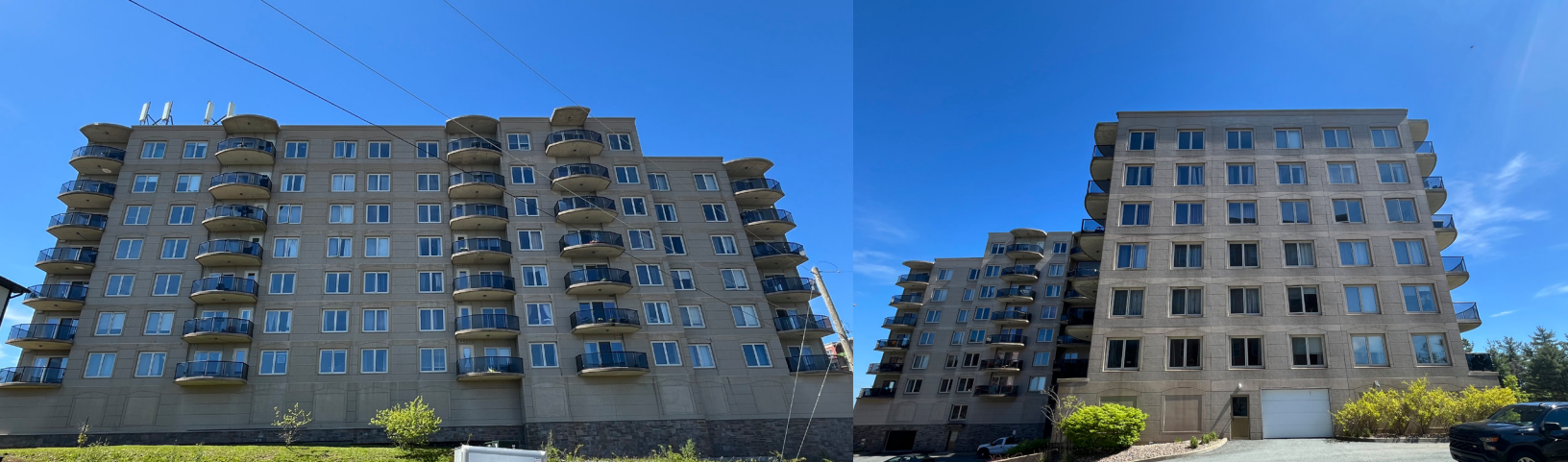
Figure 5-6: 7-storey precast concrete and cast-in-place hybrid structure used for this LCA study.
